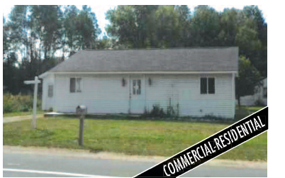
502 MAPLE, EAST JORDAN Although zoned C-1 for small business, this was previously used as a home and City says can still be. Detached garage with gas heater and a large corner lot! Very convenient location. Close to grocery store, schools, community park and downtown. Additional parcel in back is also available which provides room for a pole building. MLS 435252. Ask for Mike Stark. $49,900
