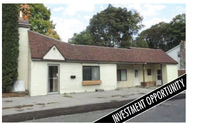
233 CEDAR STREET, BOYNE CITY Tri-plex with excellent rental history providing an opportunity for investment that is literally turn-key! All three units have had many updates making them attractive rentals. There is a 3 bed 2 bath, and two, 2 bed, 1 bath. Just two blocks from the Harborage Marina and close to downtown, MLS 435092. Ask for Jennifer Burr. $154,900
